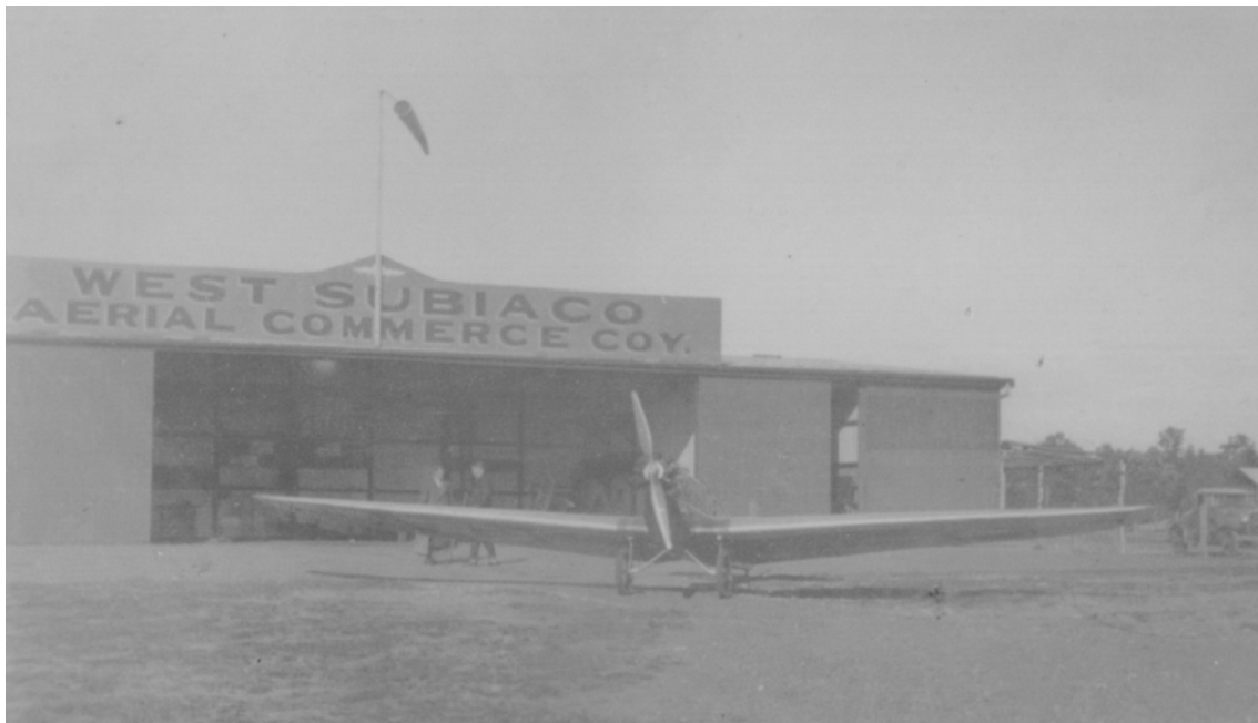
Aerial Commerce's hangar and aircraft at the West Subiaco Aerodrome c.1932
